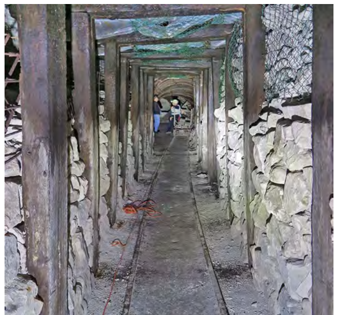
Shored-up tunnel in La Targette
